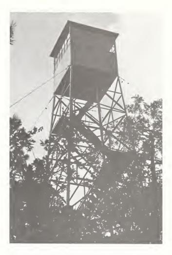
Figure 134. Lee Butte lookout, an International Derrick type built in 1933 on the Coconino.
